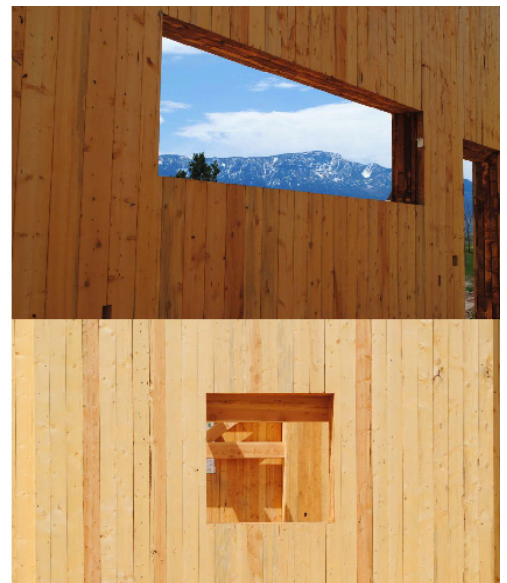
ICLT Wall Assembled and Installed On-site.
