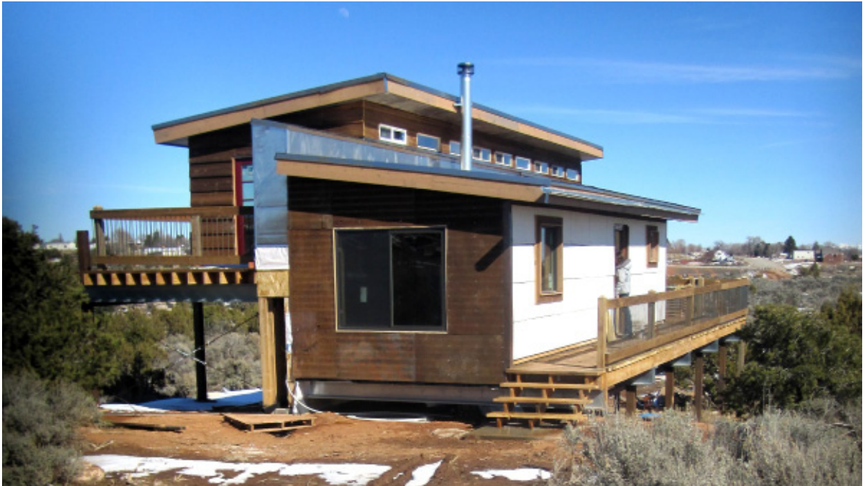
West Water House Construction
